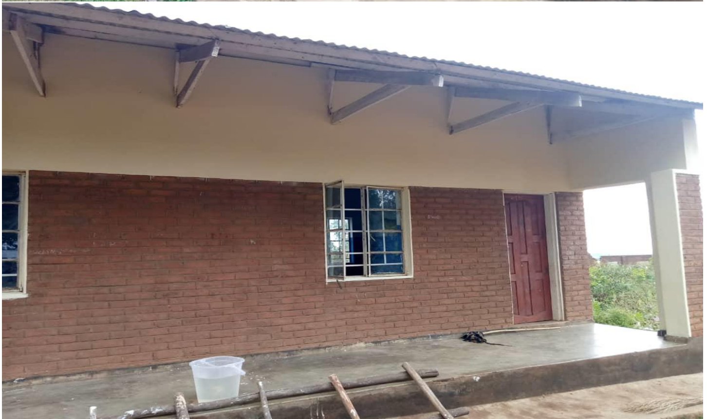
Repainted Mdumu School before having the pictures drawn.
